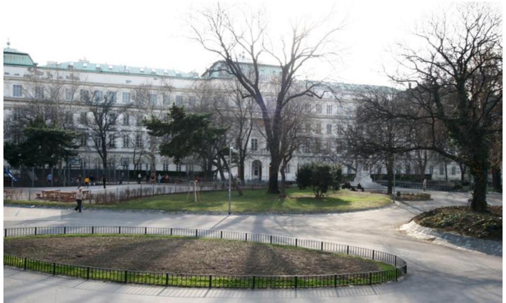
Figure 1: Vienna University of Technology – main building.
